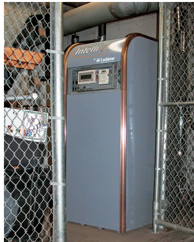
The compact physical space for both the Intelli-Fin® and the flue system made this a challenging specification.
